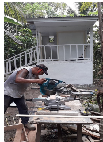
Buada District—Compost Toilet CJ Construction at work.
